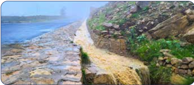
A rural road in Al Mahweet post-rainfall, showcasing effective drainage and erosion control.
